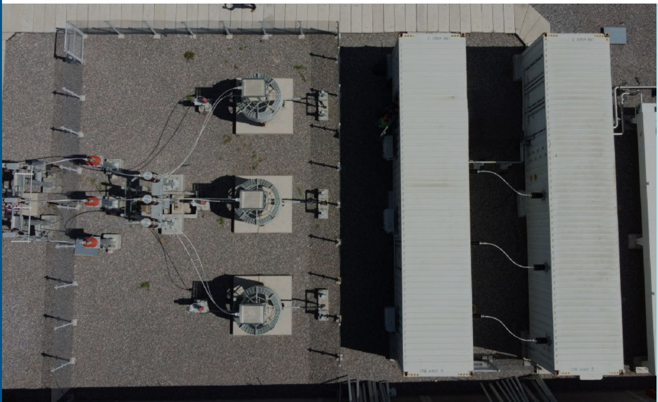
Figure 4. Upgrading 80 Mvar SVC with 40 Mvar STATCOM
