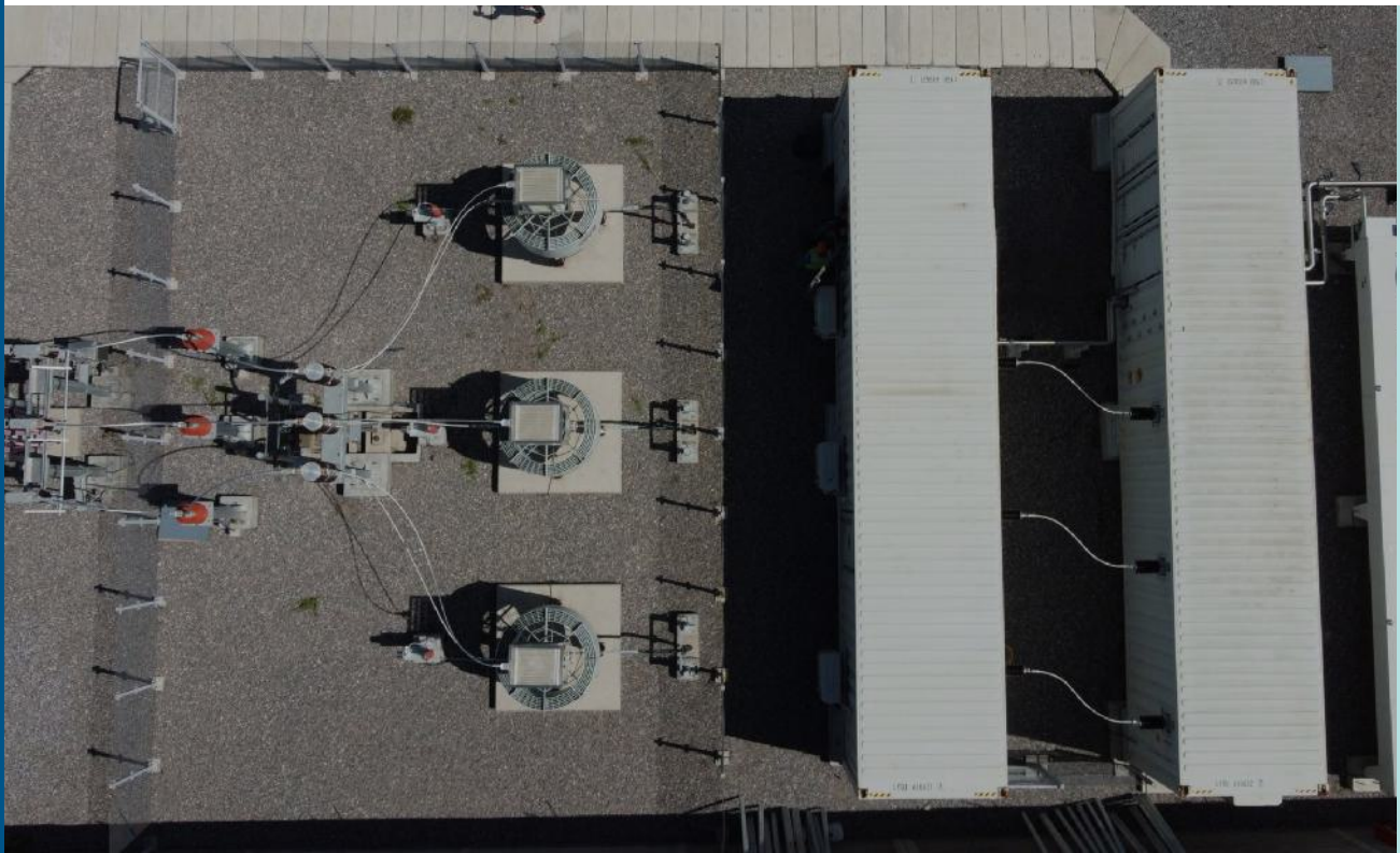
Figure 4. Upgrading 80 Mvar SVC with 40 Mvar STATCOM
