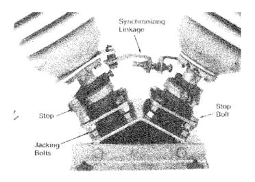
Figure 3: Rotating Insulator Bearing Housing
