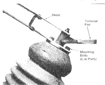
Figure 2: Live Parts Mounting
