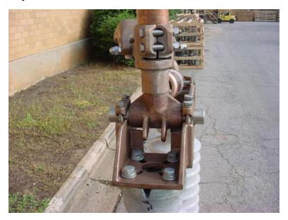
Figure 7: Typical Operating Mechanism
