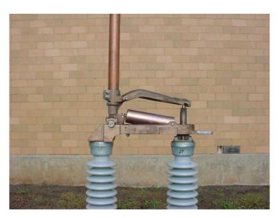
Figure 3: Stack Insulators
