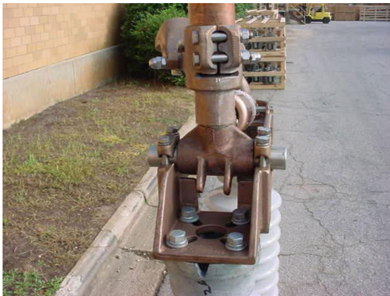
Figure 7: Typical Operating Mechanism
