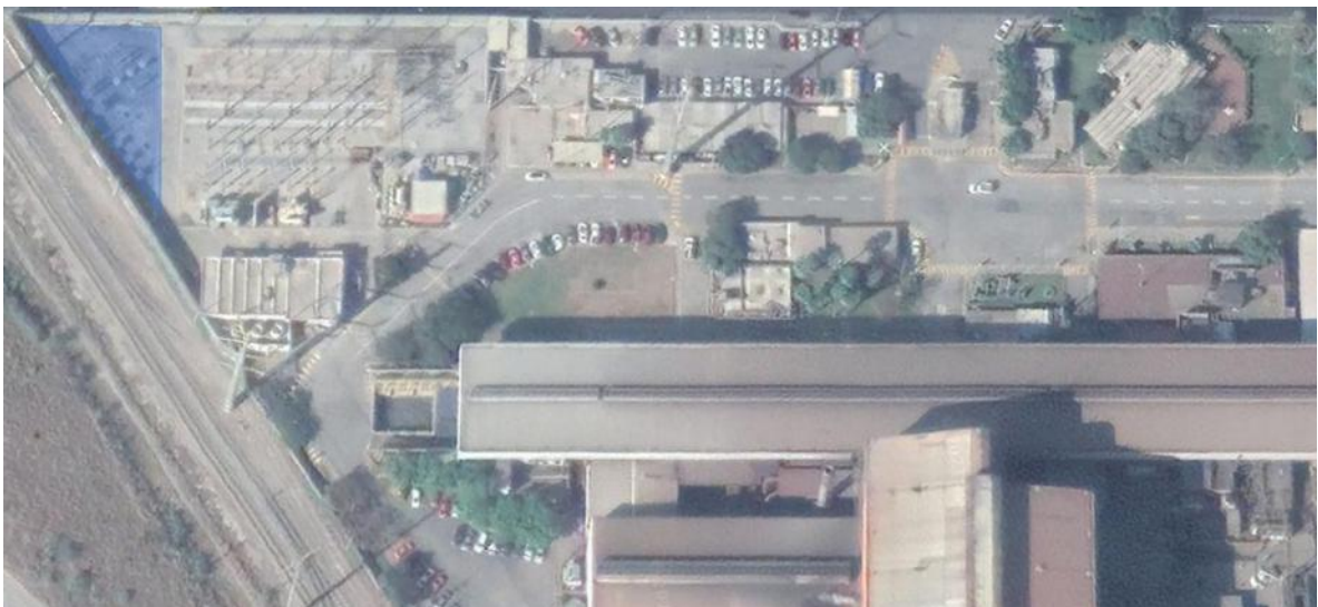
Aerial view: Highlighted in blue is the available space for the STATCOM solution with the previous harmonic filters.
