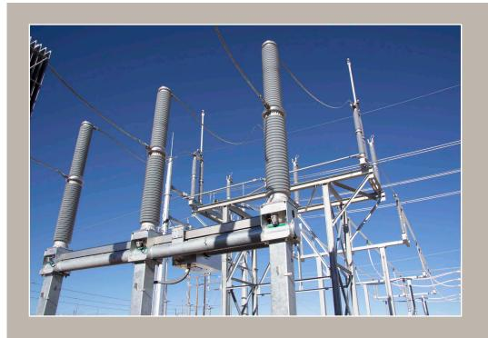
Vertical Interrupter Circuit Switcher Powered by MEPPI 245 kV
