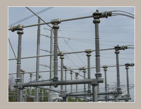
RDA Heavy Duty Aluminum Double End Break Switch
