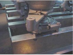
Figure 6: Bearing Stops
