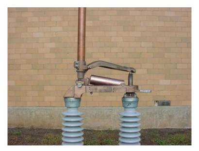
**Figure 3: Stack Insulators**
