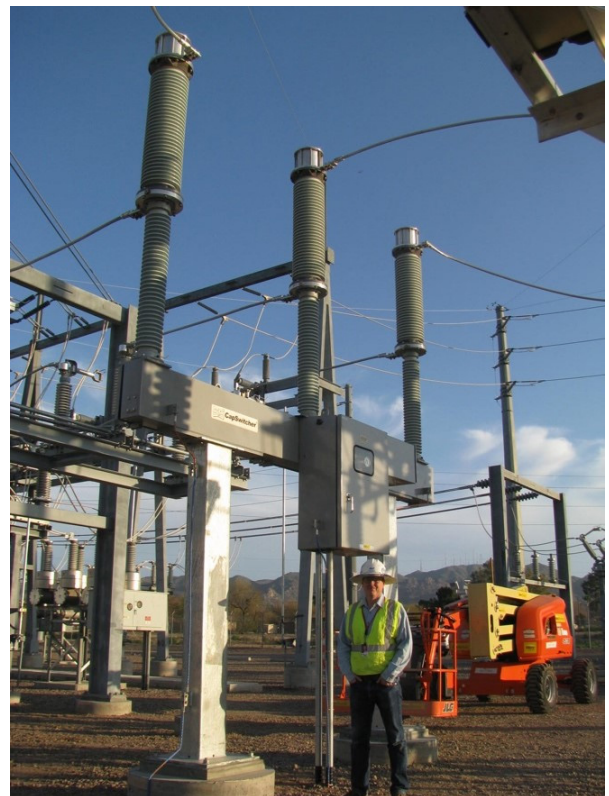
Professional Electrical Engineer Andy Keels with Salt River Project's latest 69-kV, 40 kA CapSwitcher® , located in a residential area.
