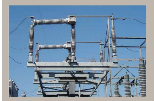
CSH2 & CSH2-B Horizontal Interrupter Circuit Switcher 38 kV – 145 kV
