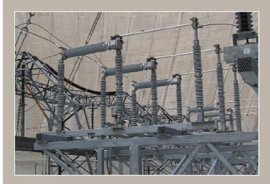
CSH & CSH-B Horizontal Interrupter Circuit Switcher 245 kV
