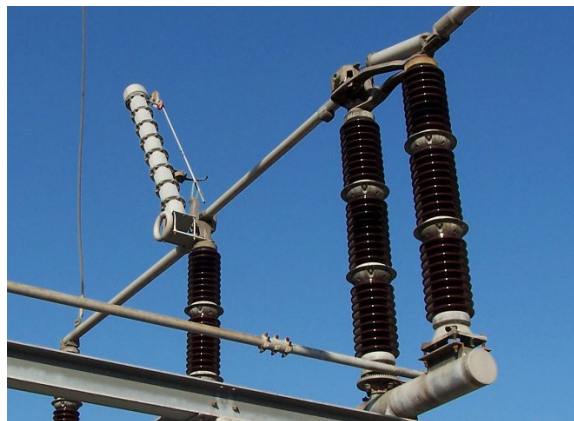
Fig. 2. Typical 145 kV Vacuum interrupter, requiring six individual bottles in series.
