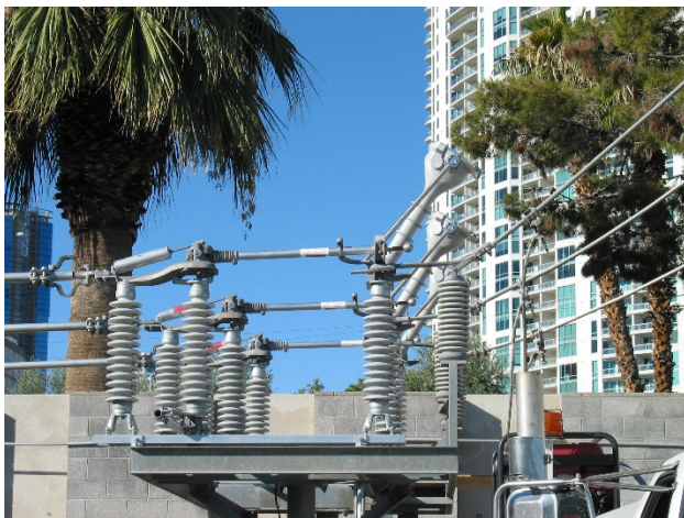
Fig. 6. 72.5 kV SF 6 single-gap attachment.
