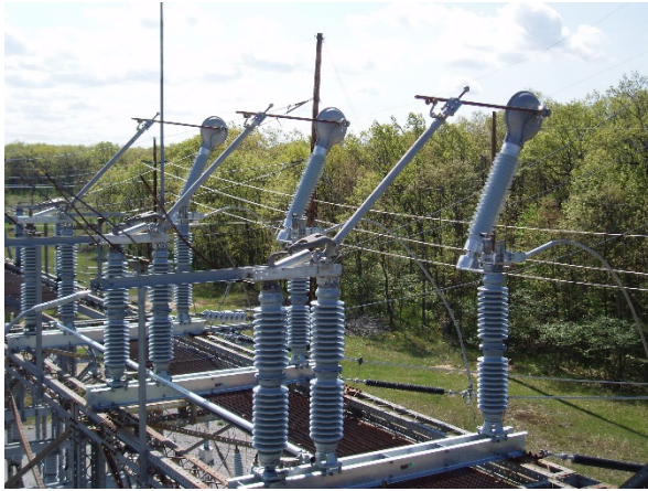
Fig. 5. 145 kV 2000A SF 6 Load Break Switch.
