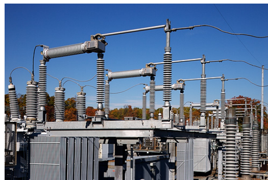
Fig. 3. 121kV Circuit Switcher (In-series) interrupter.
