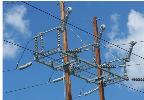
Fig. 7. 145 kV Load Break Switch on tall Wood Poles.
