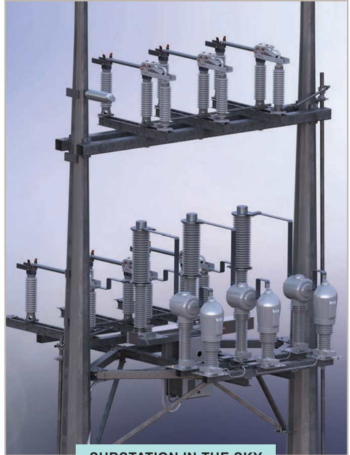
SUBSTATION IN THE SKY
