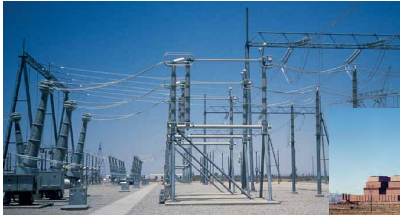
500 kV EV vertical break disconnect.
