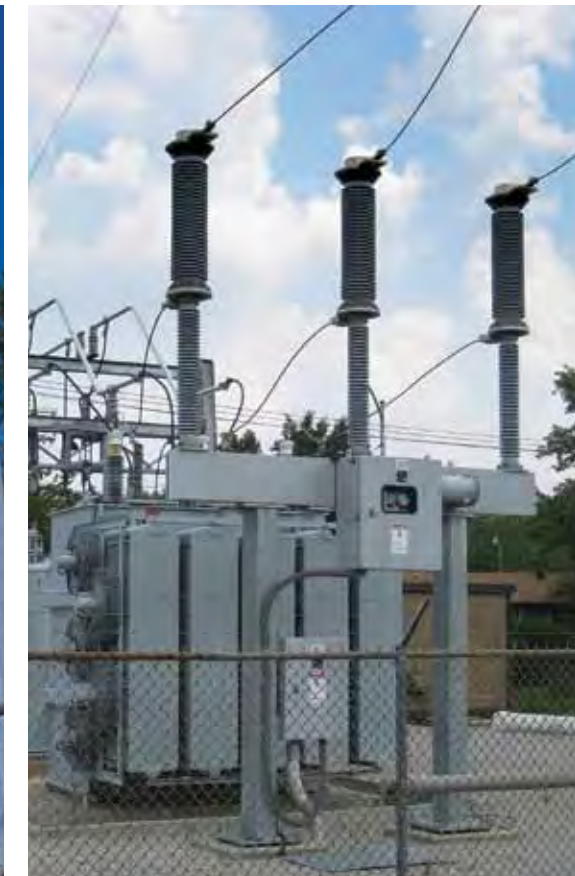
72 kV CSV Circuit Switcher.
