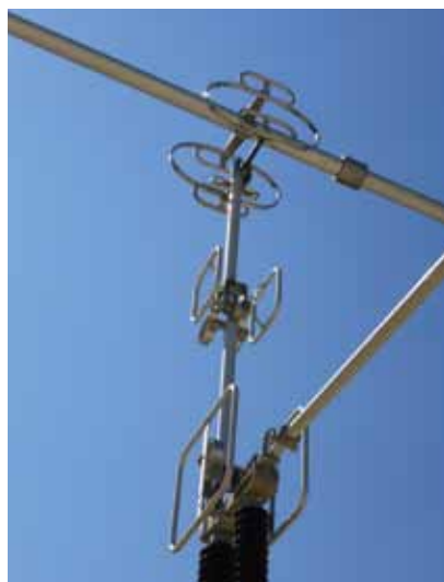
Type SPP semi-pantograph disconnect.
