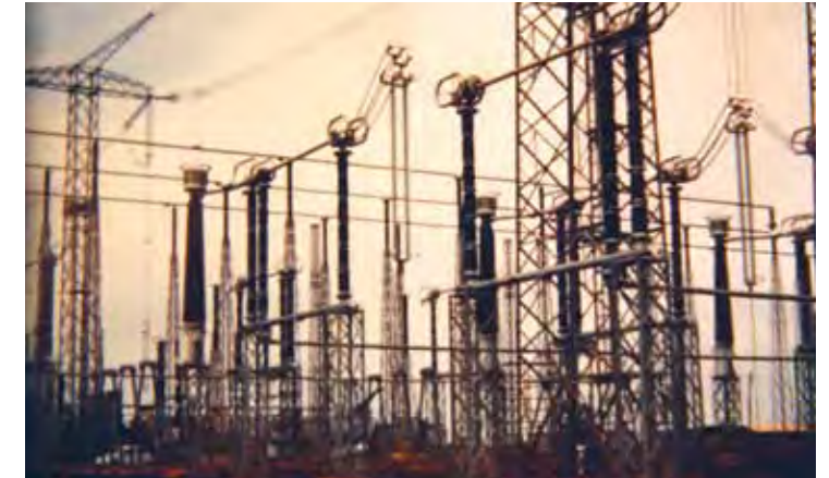
800 kV type EV Disconnect at Itaipu Dam.
