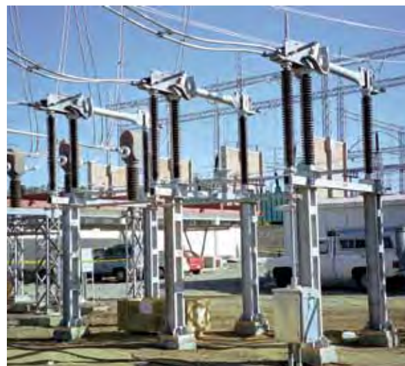
Type SLOB vertical break disconnect.
