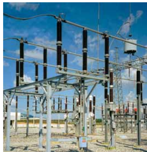
Type TCB double break disconnect.
