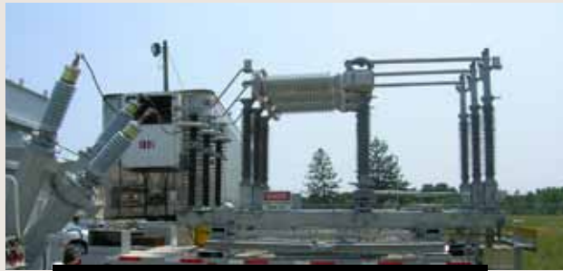
CSH-B all composite interrupters, support insulators and lightning arrestors
