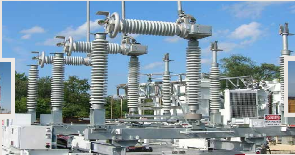
145kV CSH-B with racking mechanism on a custom tag-along trailer
