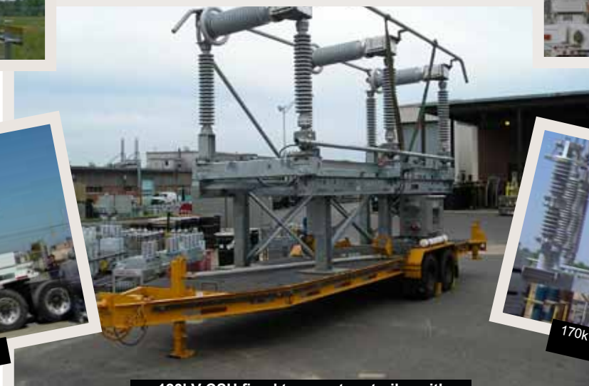
123kV CSH fixed to a custom trailer with remote control box
