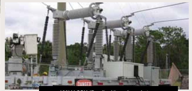
123kV CSH (fixed) with on-board stage
