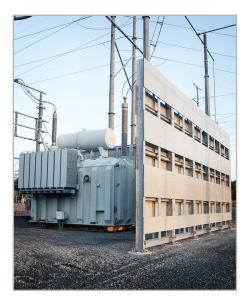
Each ballistic panel is fire rated for one hour per ASTM E-119-09c Fire Tests of Building Construction & Materials. Panels meet Flame Spread Rating of 45 and Smoke Development Rating of 165 per ASTM E-84-08a, "Standard Method of Test for Surface Burning Characteristics of Building Materials" achieving NFPA & IBC Class A & B Fire ratings.
