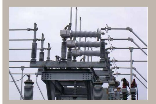
LSH & LSH-B Horizontal Interrupter Line Switcher
