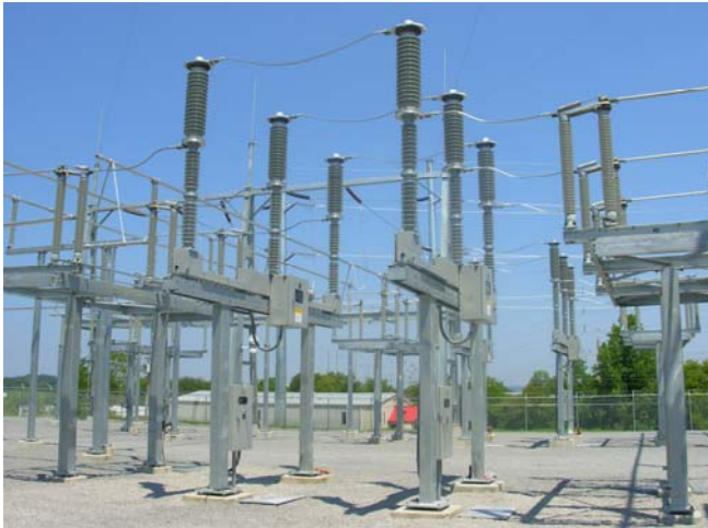
Goose Creek Substation (Circuit Switcher with local, series connected interrupter)
