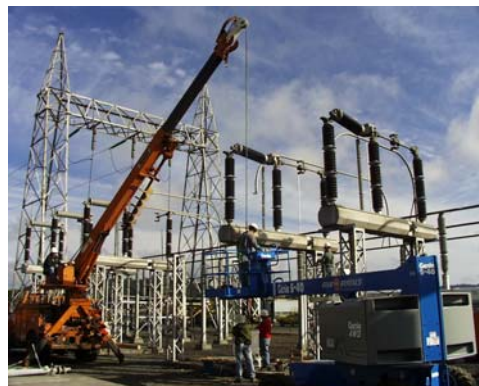
Existing Circuit Switcher Removed
