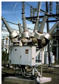
Circuit Breakers
