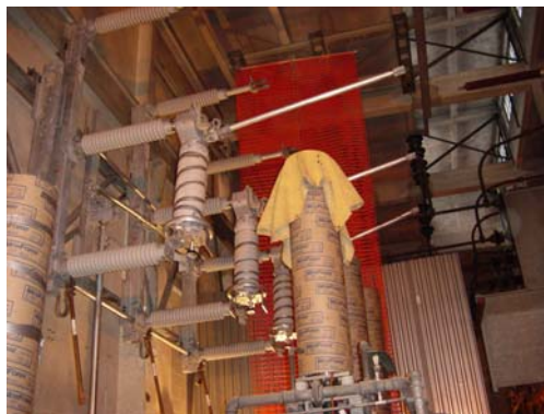
New Southern States LSH-B being installed
