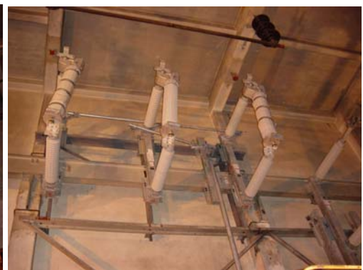
New Southern States LSH being installed
