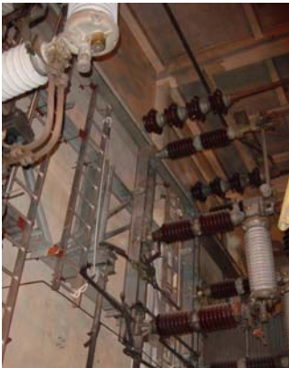
One of the old competitor's units being replaced
