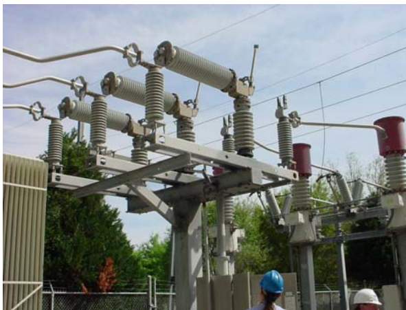
Before: The failed competitor's circuit switcher
