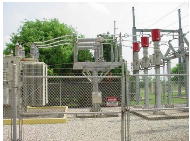
After: A fully functional and energized Southern States CSH-B
