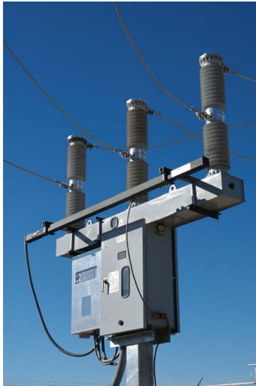
Figure 7 Reactor Switcher Equipped With Three-Phase Non-Contact Non-Saturating Current Transformer
