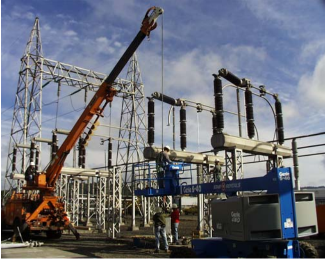
Figure 9 – Shows a competitor’s circuit switcher being removed from its support structure.
