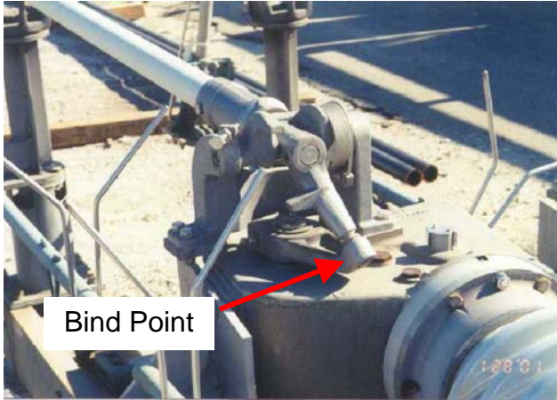
Figure 6 – “Dog leg” style hinge
