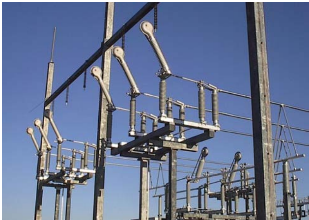
Newest Single Gap Per Phase SF 6 Interrupter On A Vertical Break Switch (2003-Present SF 6 Interrupter) Figure 4
