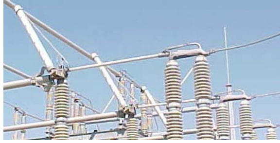
Multi-Module Per Phase Vacuum Interrupter On A Vertical Break Switch Figure 3
