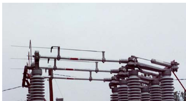
Quick Break Whip Type Arcing Horns On A Vertical Break Switch Figure 2
