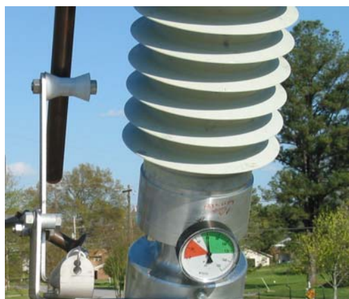
Close Up Of SF 6 Interrupter's Color Coded Pressure Gauge (Needle In Green Range As Shown Indicates Adequate Dielectric Is Present For Successful Interruption.)
