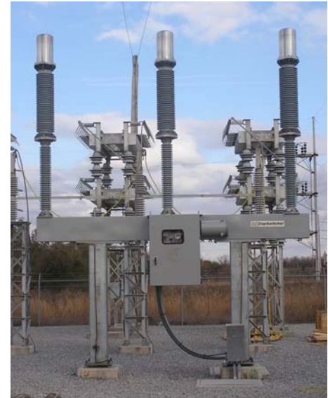
72.5 kV CapSwitcher ® with closing resistors shown at left.
