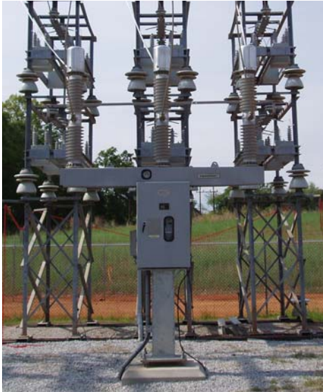
72.5 kV CapSwitcher ® with closing resistors shown at left.
