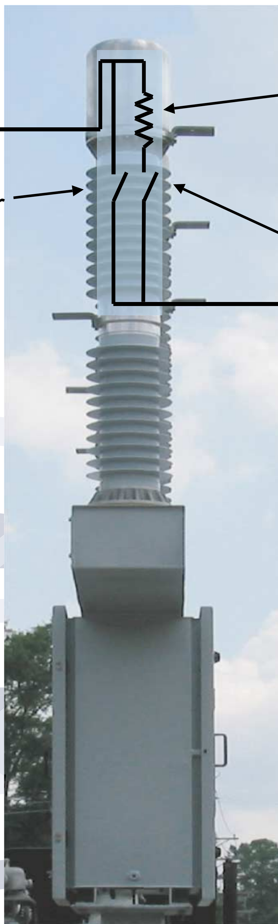
Closing Resistor
